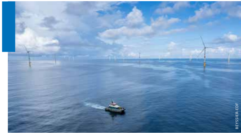
Saint Nazaire Wind Farm (480 MW) has been up and running since 23 November 2022, and is the France's first commercial offshore wind farm, equipped with eighty General Electric GE Haliade 160-6 MW type wind turbines.
