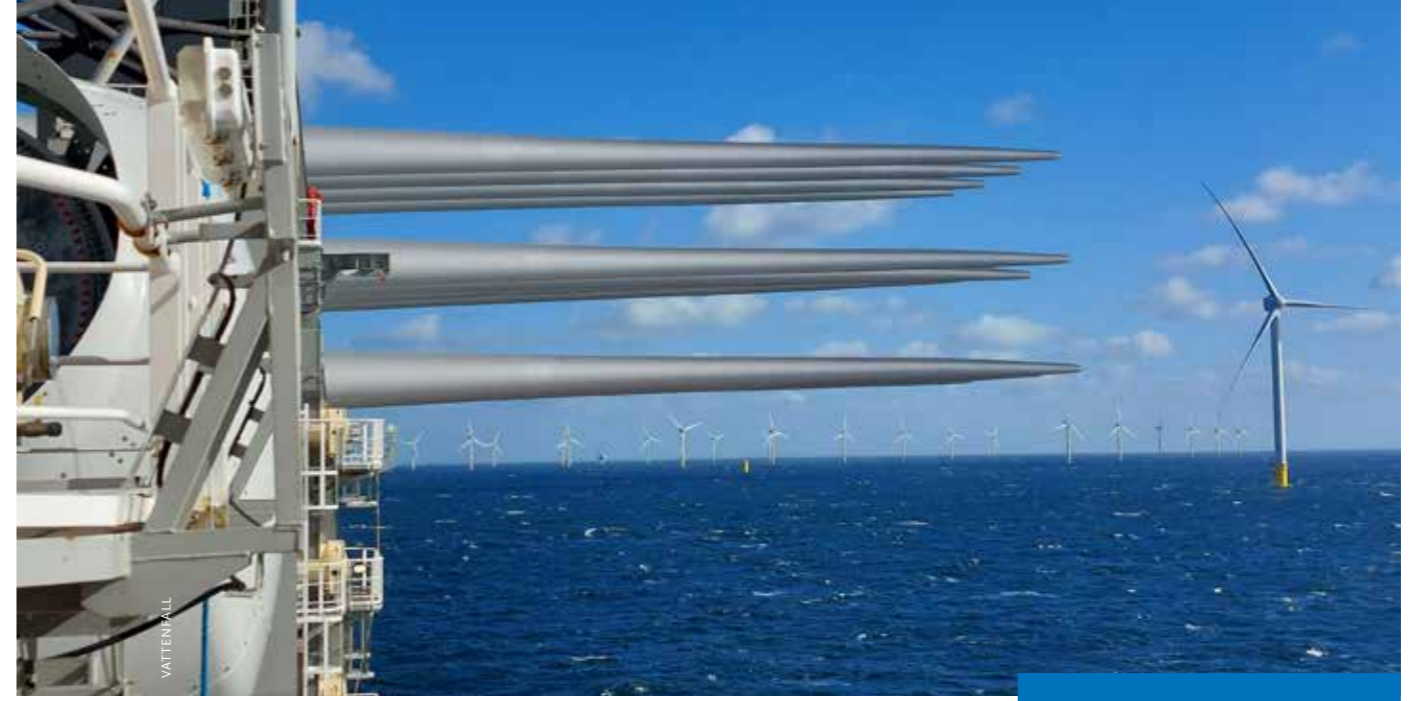
The Netherlands’ Hollandse Kust Zuid 1&2 Wind Farm is the world’s first unsubsidized offshore wind farm.
